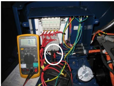
The resistance test checks if there are any shorts or opens in the winding:
